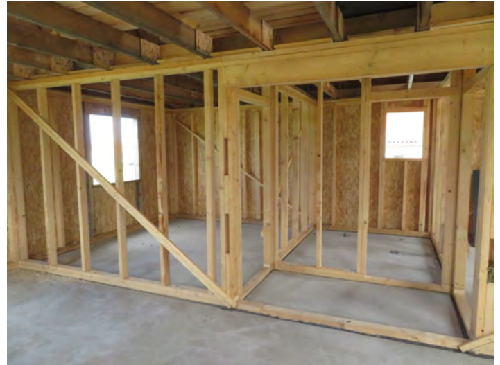
Above: The interior of the house well under construction.
