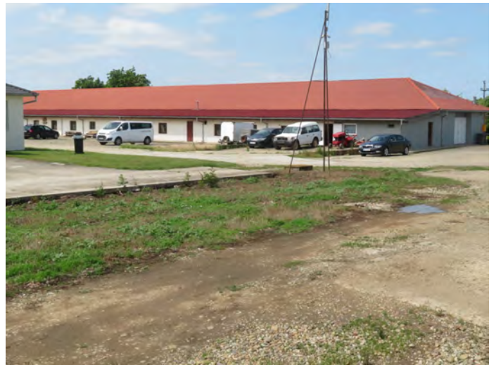
Above: The extensive area housing various trade workshops.
