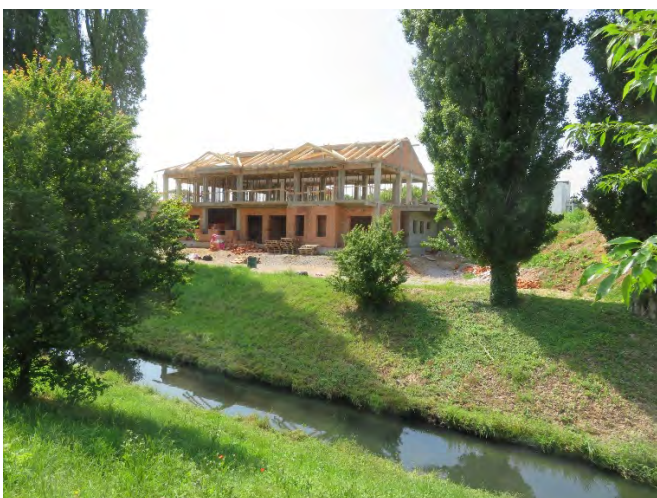
Above: The new hospice building is progressing well.
