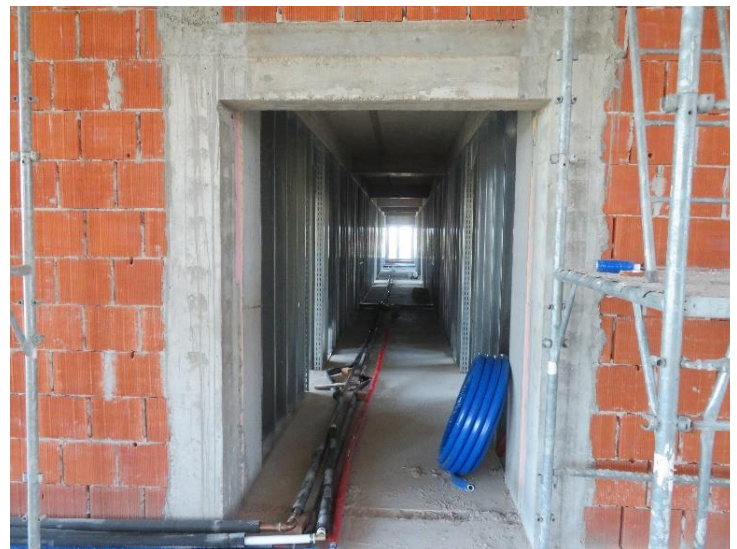
Above: A view of the corridor as the building nears completion.
